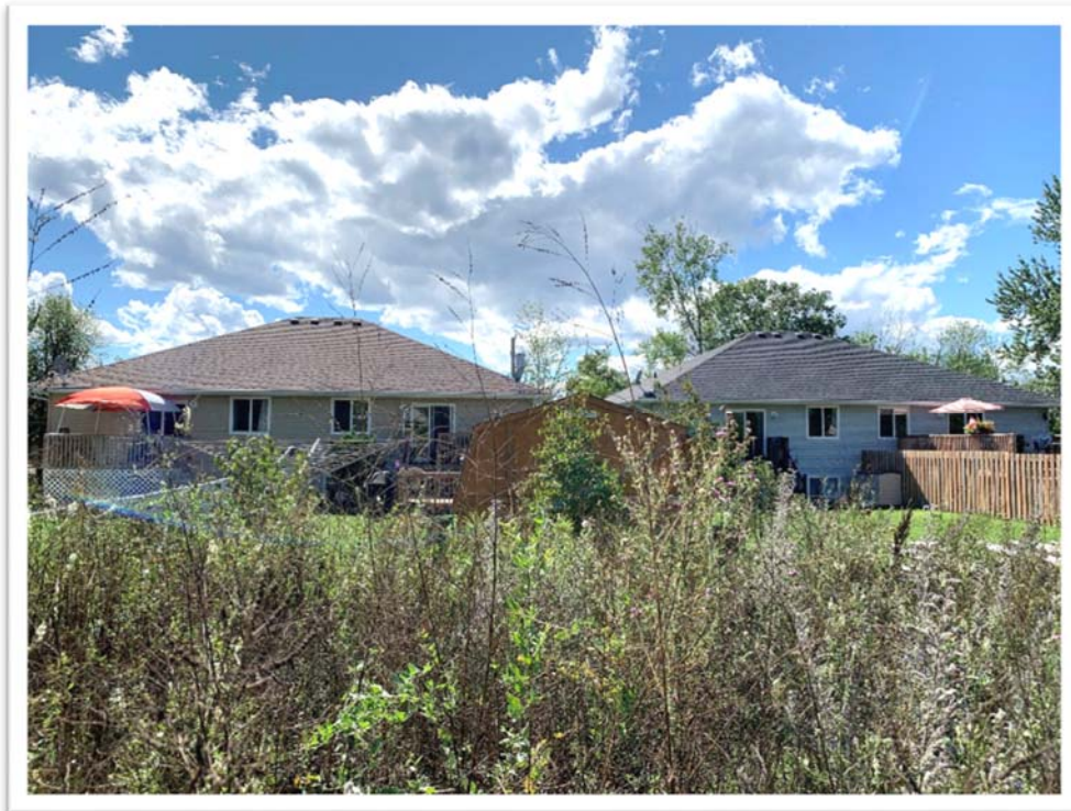
Subject Property – View looking west from interior side yard.
