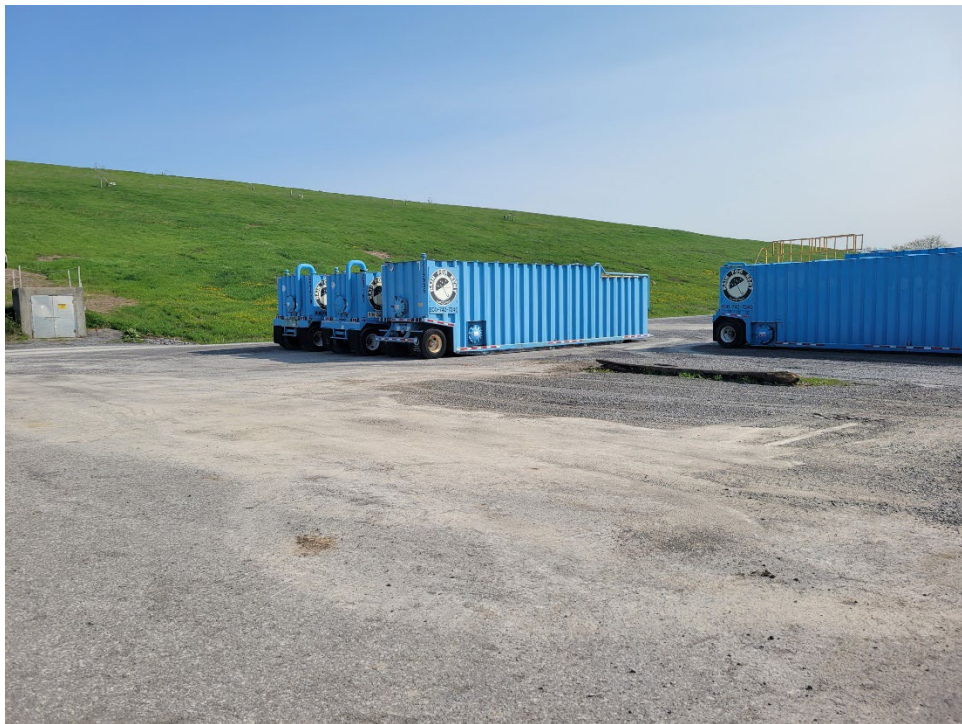
Photo 4: Site conditions following removal of impacted soil and final grading with clean gravel (May 8, 2023)
